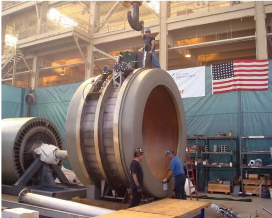
Installation of the rotor in the stator
